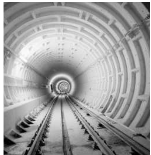
Looking east inside newly constructed TTC subway tunnel, 1968. (City of Toronto Archives)
