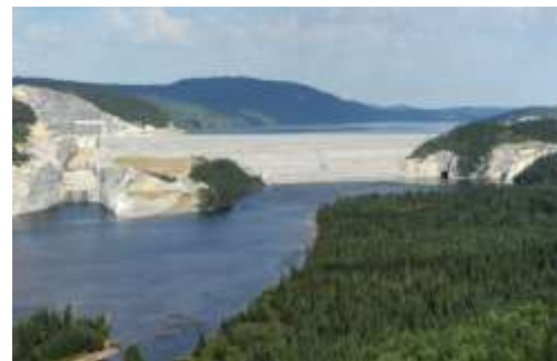
Péribonka main dam and spillway.
