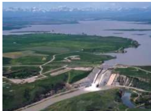
St. Mary reservoir and new spillway during a spring flood event.
