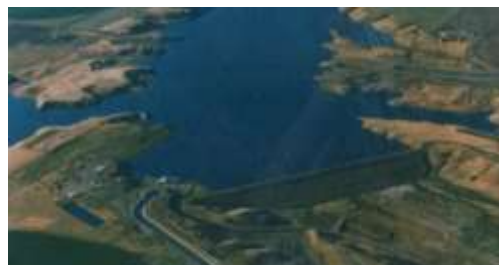
Forty Mile Coulee Dam and reservoir after completion in 1988.
