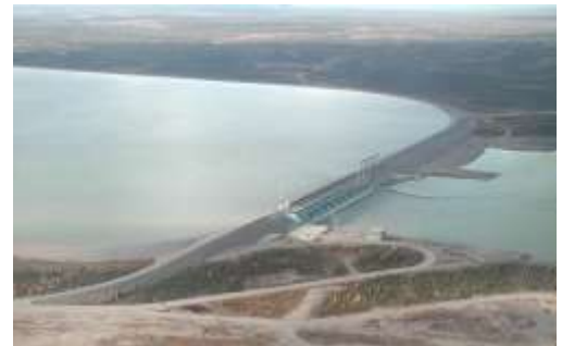
Aerial view of the Long Spruce Generating Station; dikes constructed on discontinuous permafrost extend to the upper left. Photo by Manitoba Hydro.
