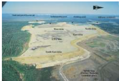
Aerial view of the LTA site before construction of the cover.
